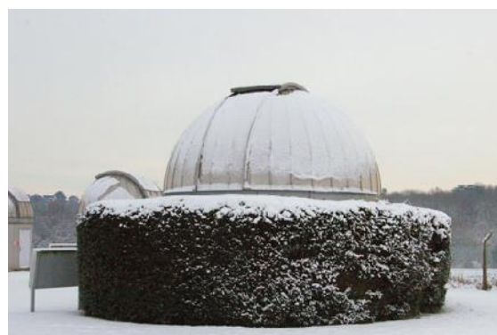
Figure 11: Detail view of the Marsh Dome (Bayfordbury Observatory).
