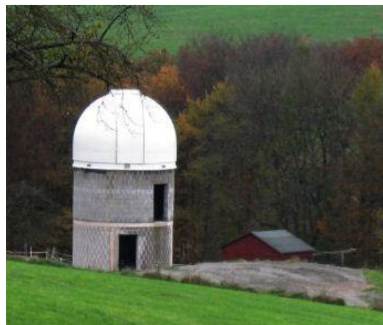
Figure 14: The body shell of the telescopic tower for the STScI main instrument (STScI).
