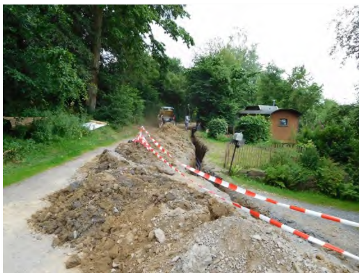
Construction of the supply channel.
