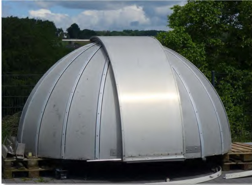
The 3.5m dome for our upper substation.
