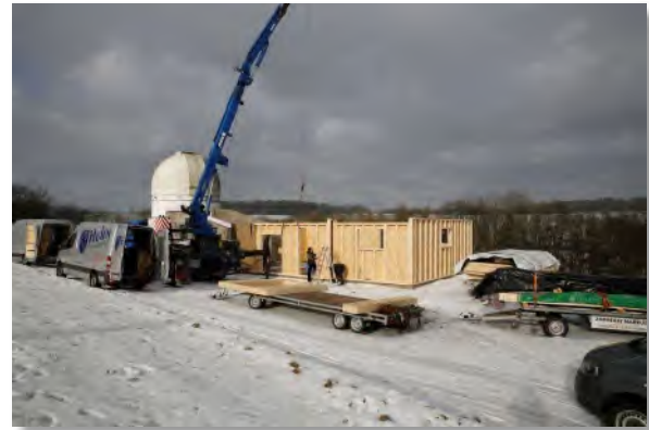
Construction of the service building.
