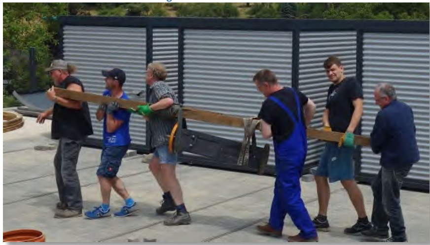
Dismantling the Bode observatory and unloading in Schnöringen.
