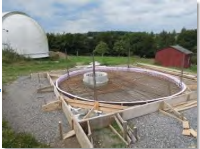
Construction of the tower base
