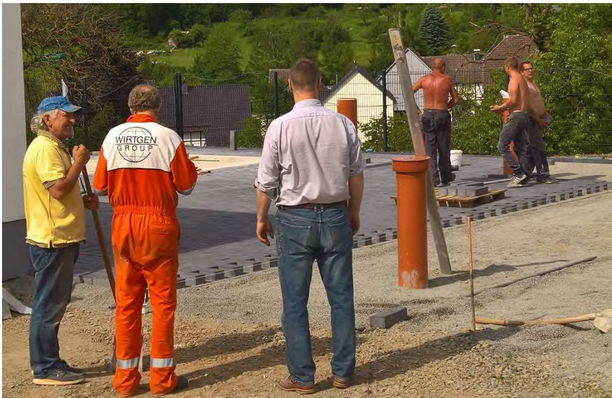
The paving is laid. Wojciech Walczak on the left.
